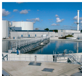
Waste water treatment
